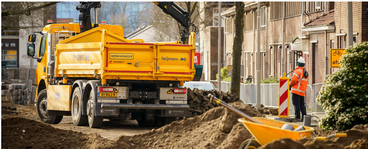
Electric truck at a project in Amsterdam
